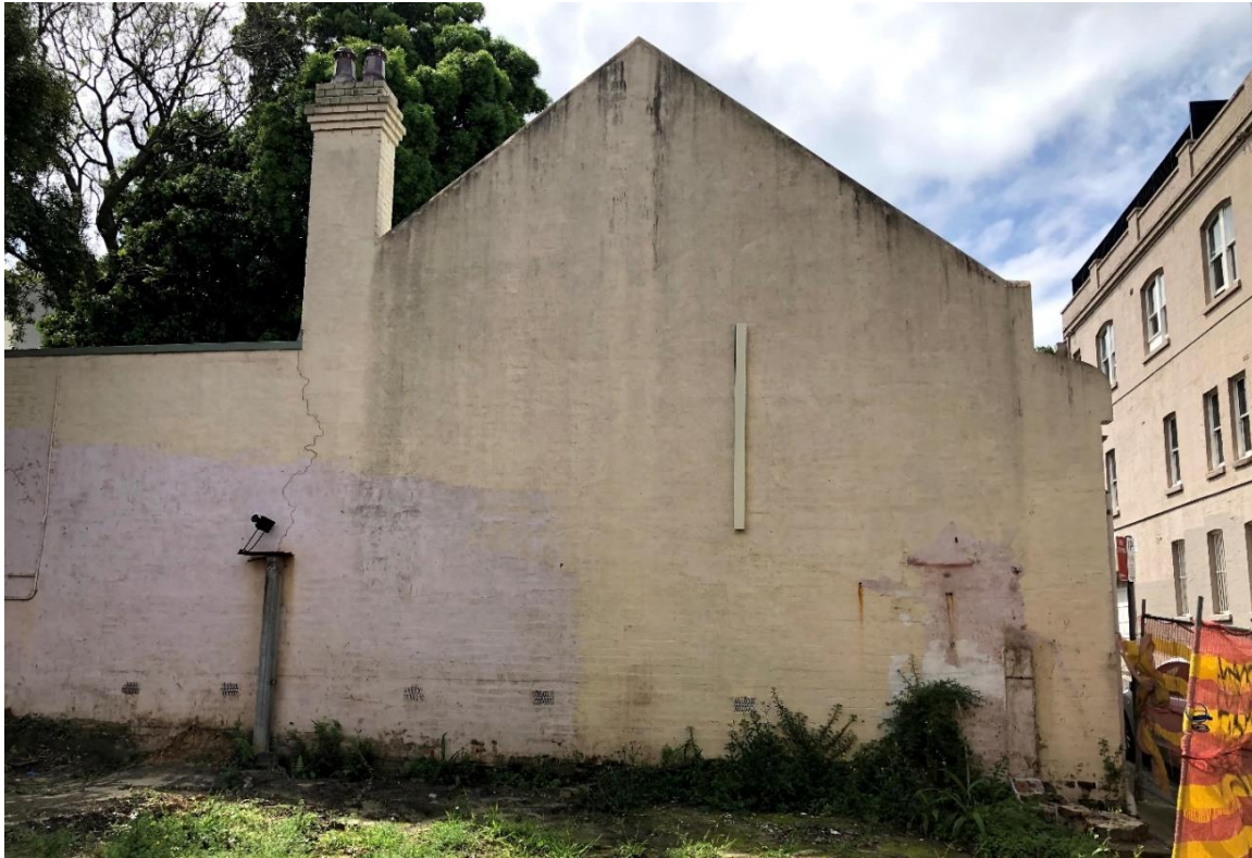
Figure 11: Adjoining site to the north: 73 High Holborn Street
