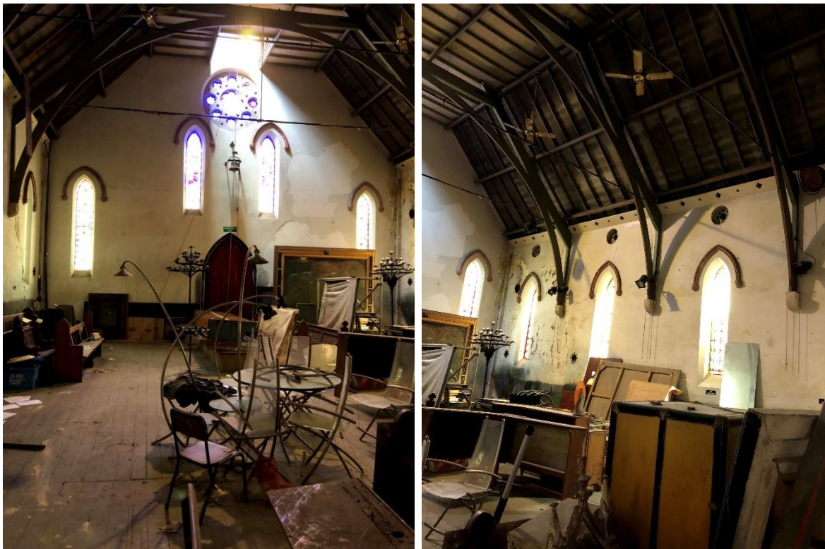
Figures 8: Building interior
