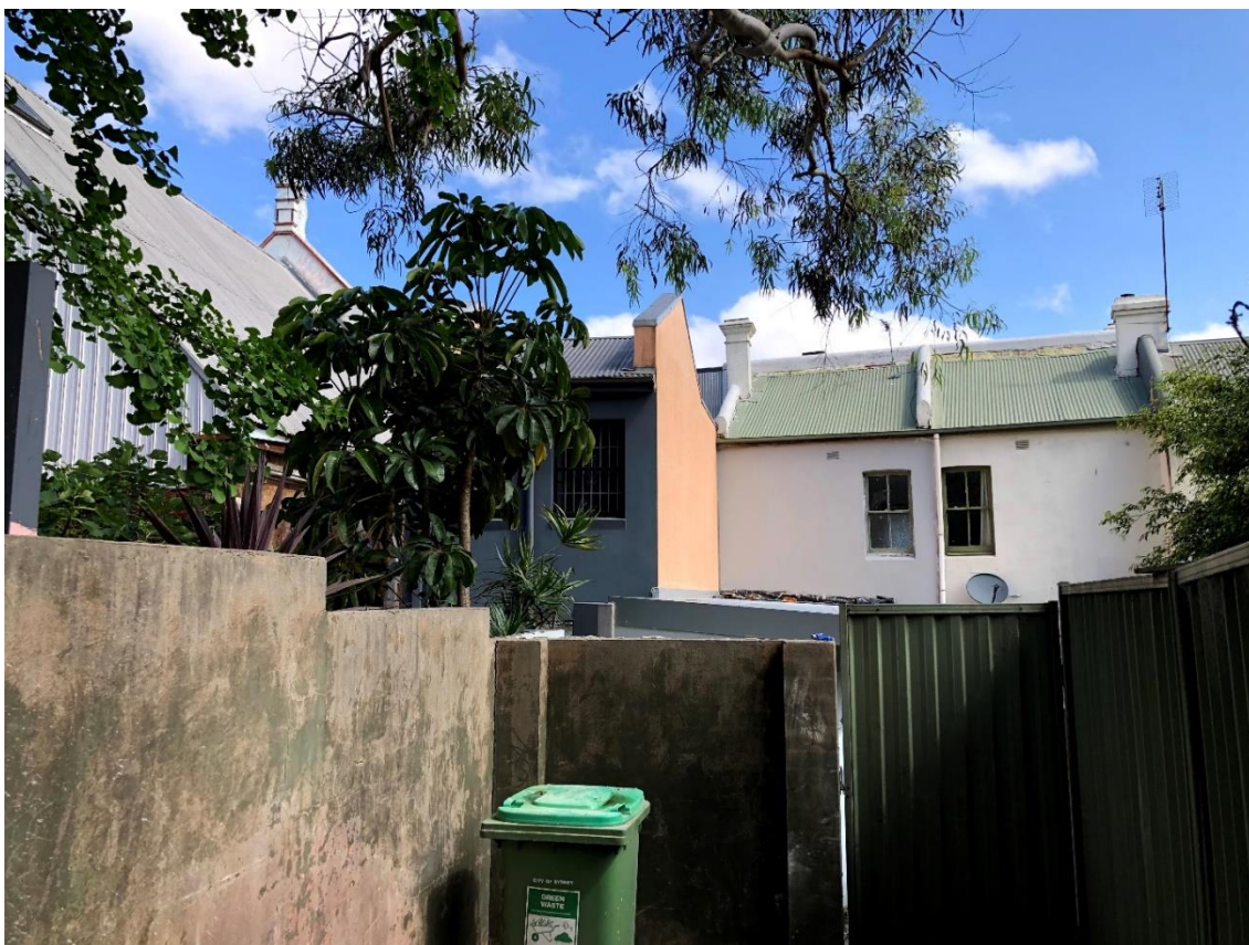
Figure 12: Sites adjoining to the west that front to Cleveland Street viewed from Goodlet Lane to the rear
