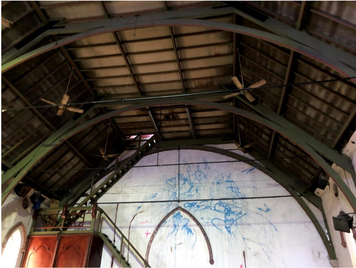
Figure 9: Building interior, northern wall
