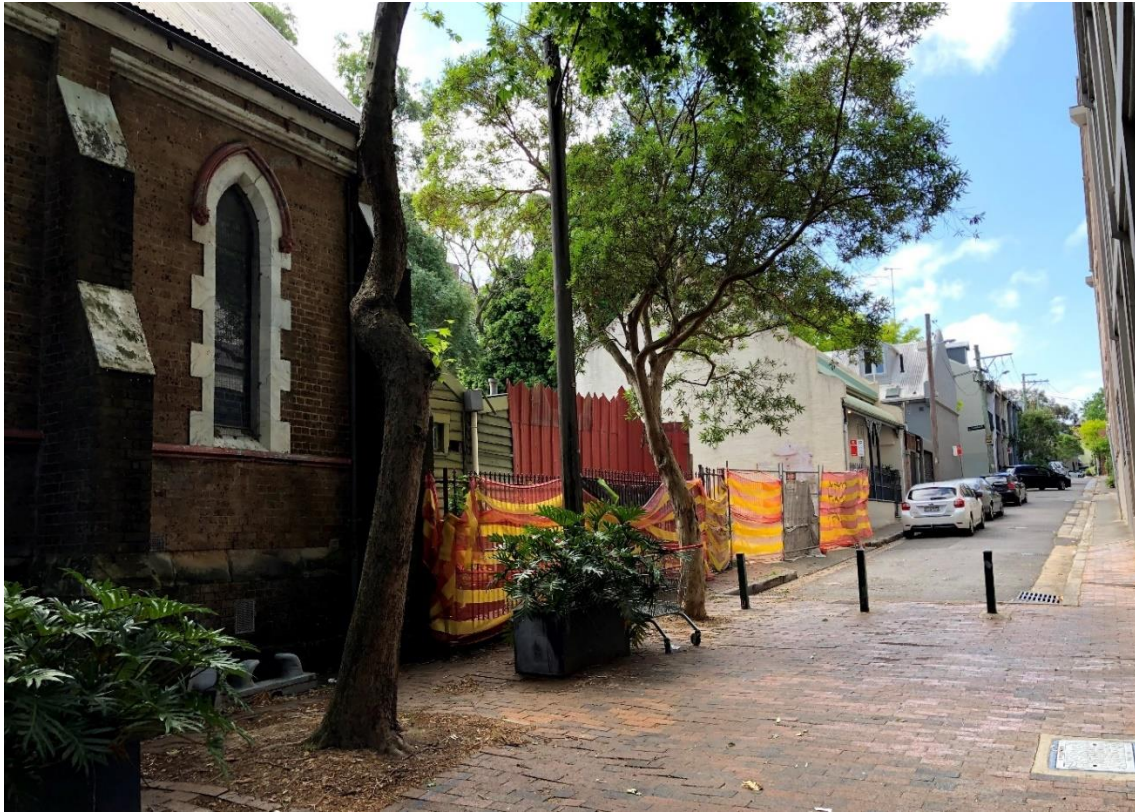
Figure 5: Site viewed from High Holborn Street looking north
