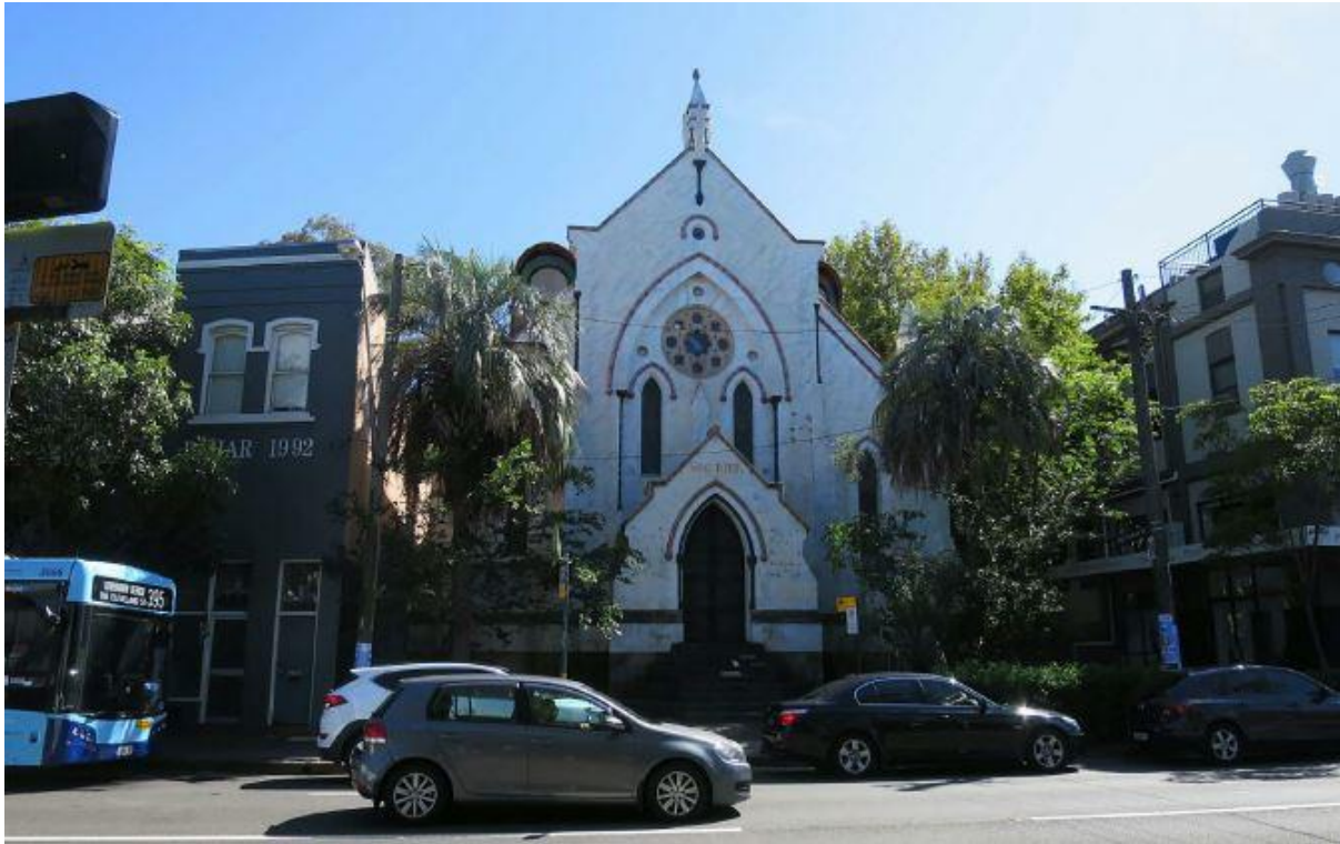
Figure 24: Montage image, Cleveland Street looking north
